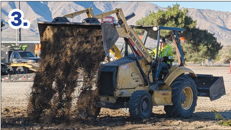
3. The grindings get spread onto the dirt.
