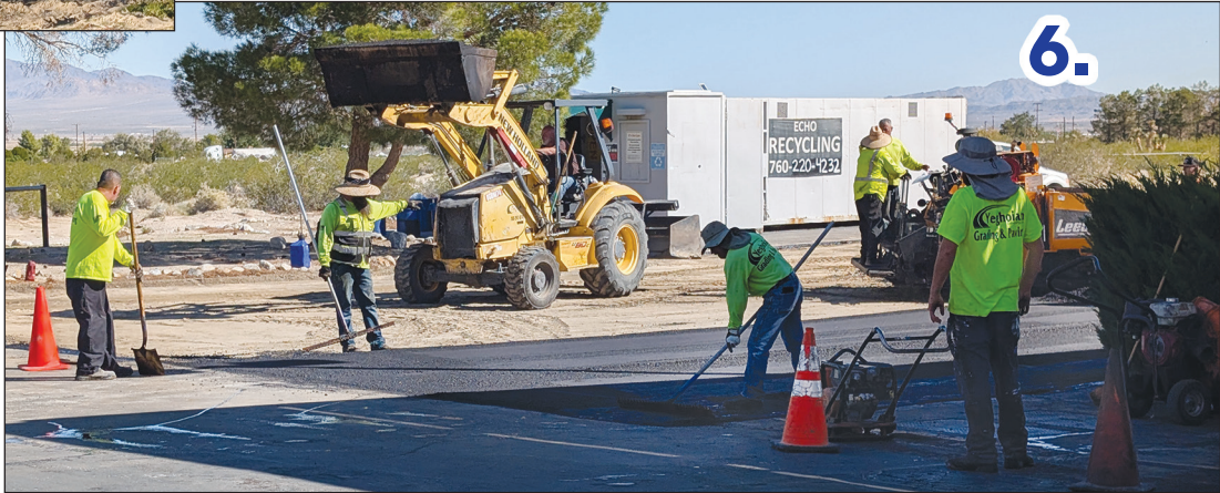
6. Even after the rolling, there is much hand work to do smoothing, making edges straight, etc. These guys really work hard !
