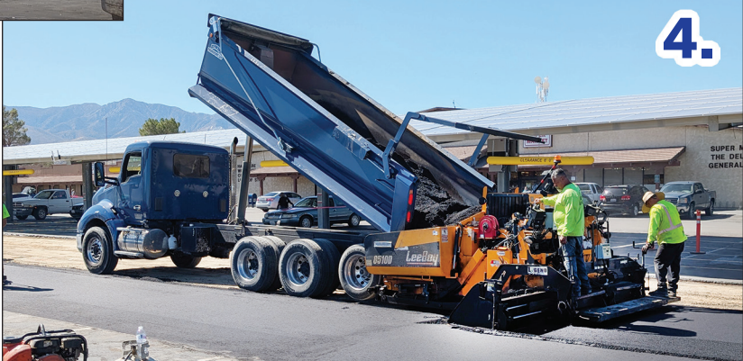
4. Trucks had to run to asphalt plant near V.V. College and bring it all the way here. Above, the truck is loading hot asphalt into paver.
