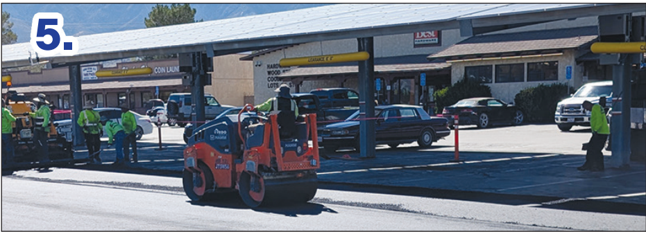
5. After the paver spreads the hot asphalt, the roller follows.
