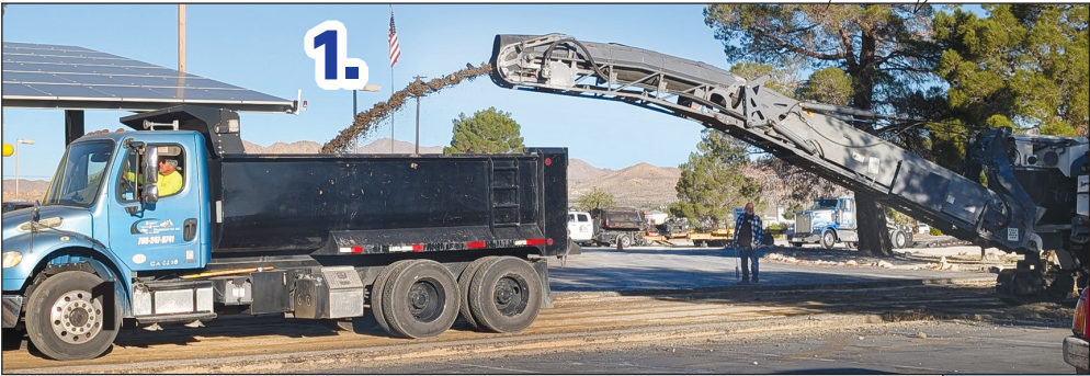
1. After a few days of crack-filling and repairs of small spots, they started the big project to replace the asphalt in the large eastern area of the parking lot. Here is the grinder at work removing old asphalt.
